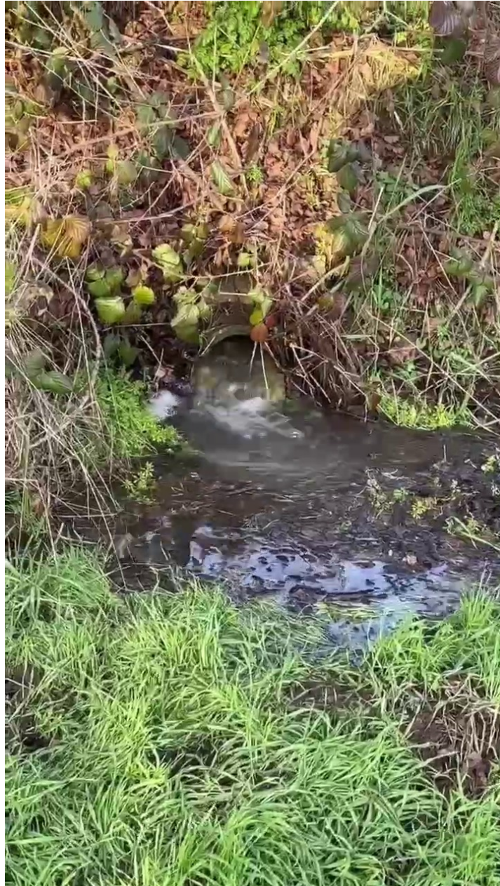
Figure 5. Water discharging from the drain-off pipe beside the footpath leading towards Maloney's. Filmed February 2026; supplied by Carole Sherris.
